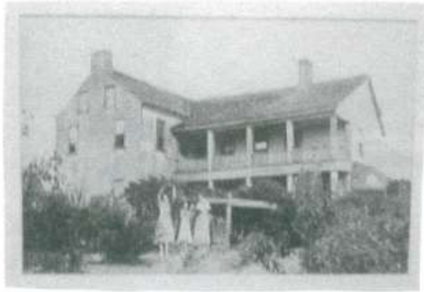
Rear addition in the late 1920's
